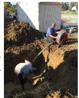
John Bedwell and Carl Williams repair a broken storm drain at Nora.
