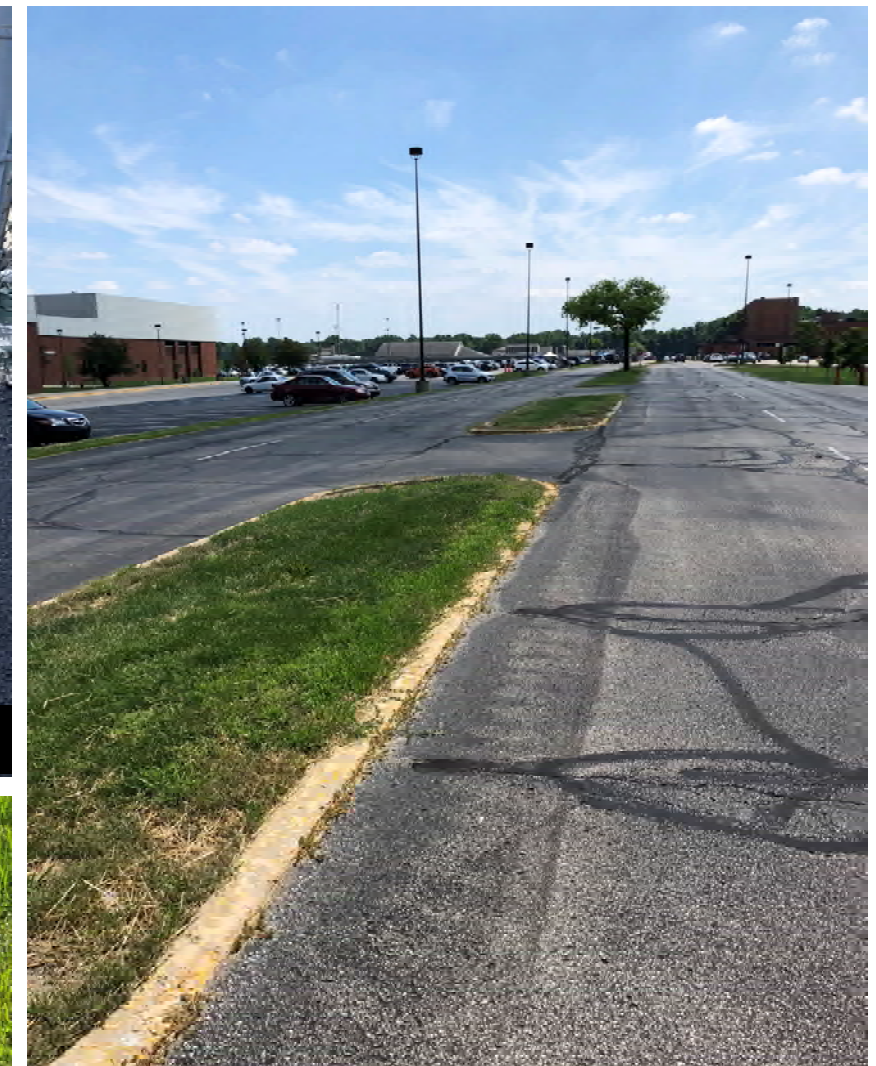
D – Curbs & asphalt - poor condition
