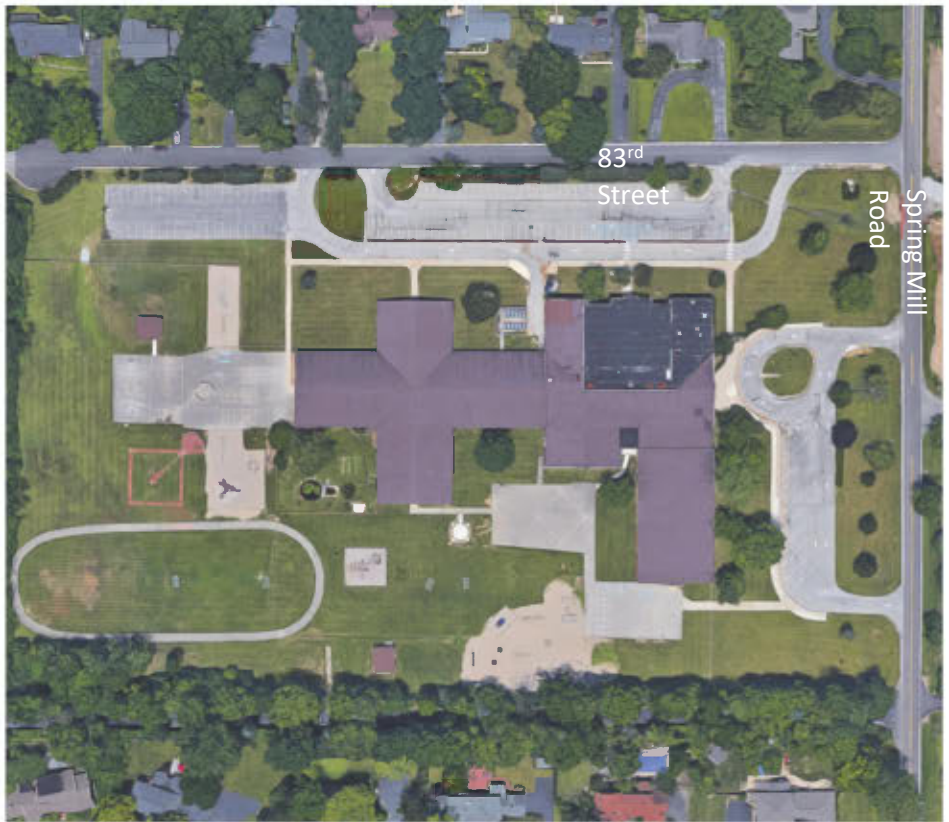
2020 proposed referendum construction scope will occur with minimal disruption to daily school operation and begin with conjunction to 2016 referendum construction scope. Majority of scope is isolated areas and exterior work.
